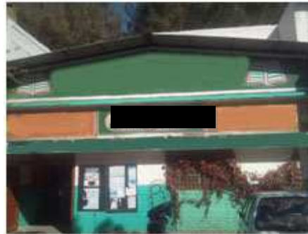
Pic 5: Face-wall of SC
