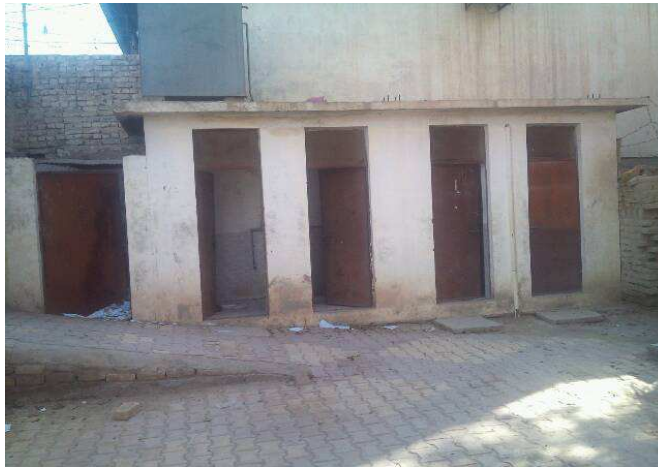
Toilet Facility at SC Quetta [Taken Date April 16 2011]
