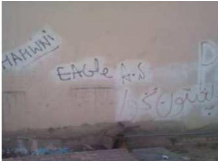
Back wall of the classroom at SC [Taken on 16/4/2011]
